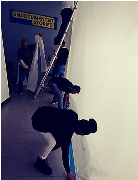
Approximately 23 day laborer recently completed U.S. EPA lead-safe certification training
